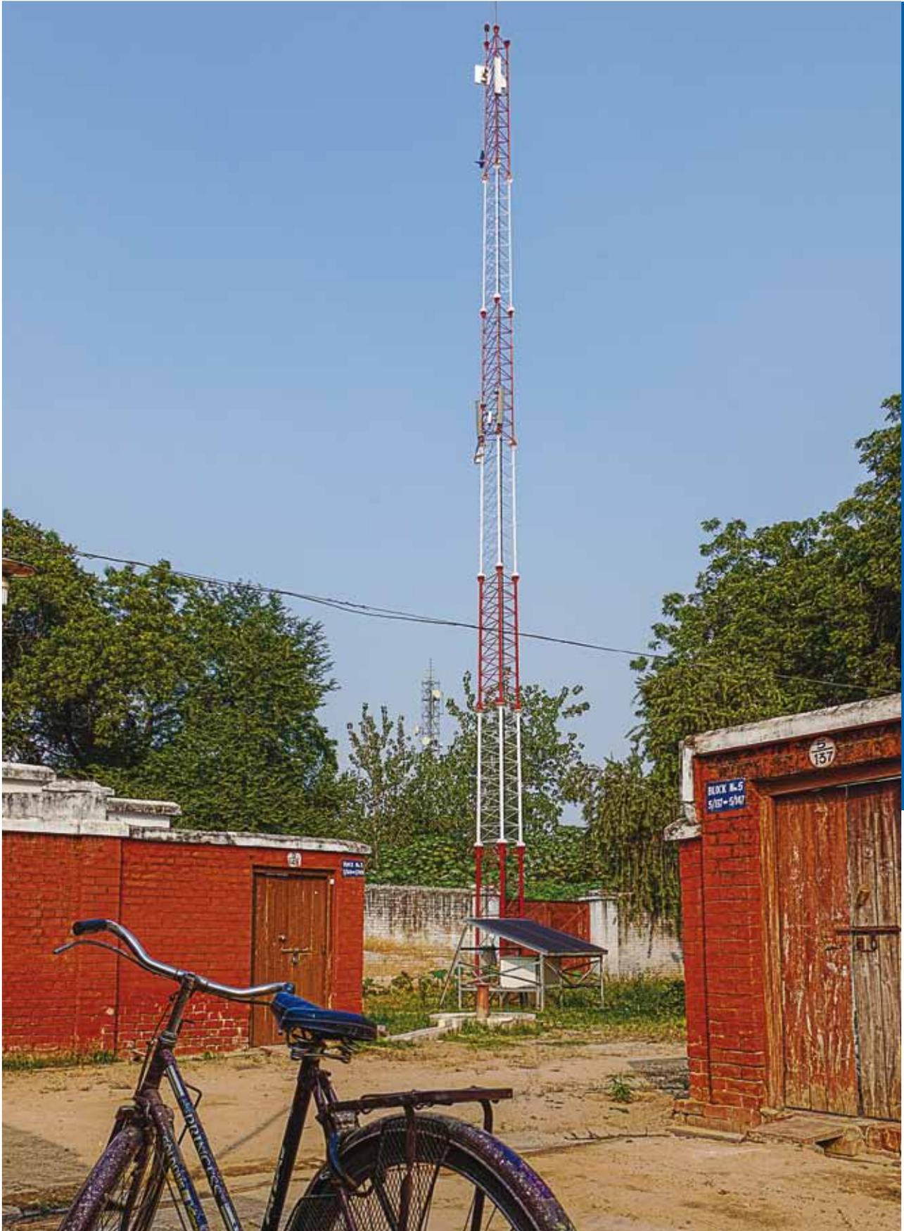
*VNL's Solar Powered 3 Sector Wi-Fi BTS Deployed at DEI, Agra, India*
