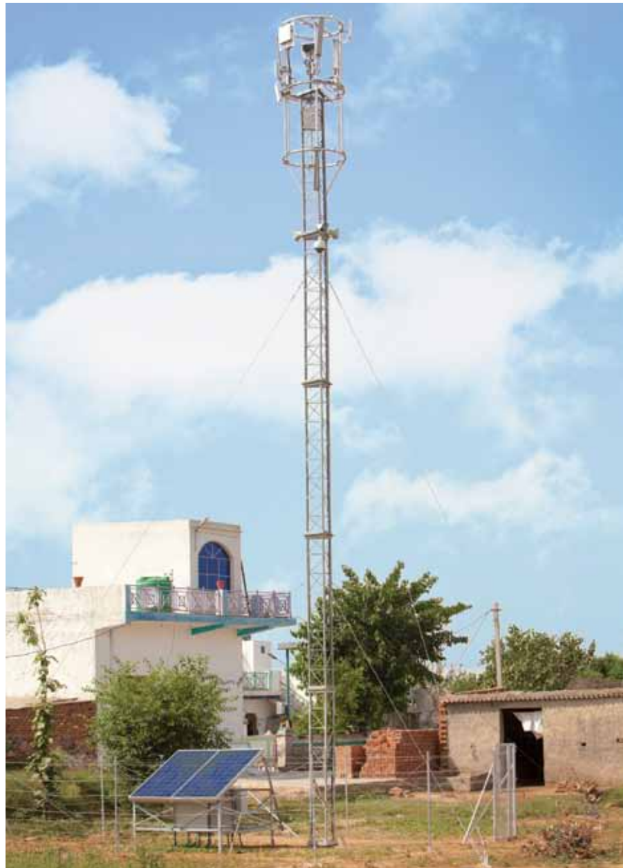
Solar-powered broadband site at Bahadari, Rajasthan
